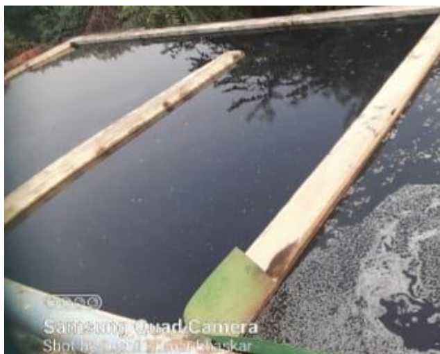
Fig. 5. Primary Settling Process (Source-Northern Eastern Railway Gorakhpur)
