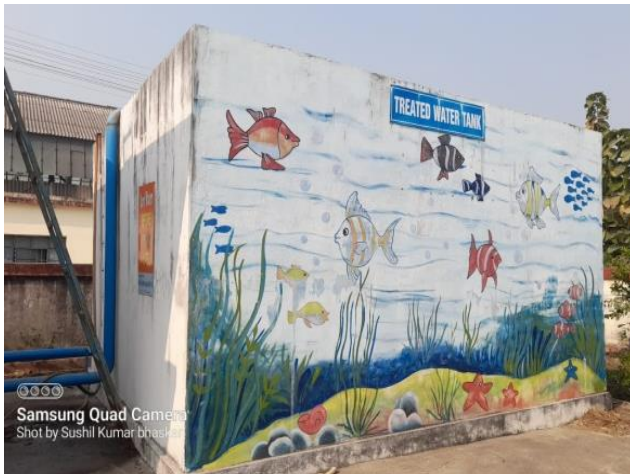
Fig. 11. Post-Chlorination Process (Source-Northern Eastern Railway Gorakhpur)
