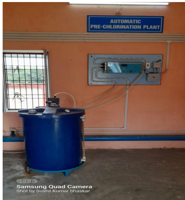
Fig. 3. Pre-Chlorination Process (Source-Northern Eastern Railway Gorakhpur)
