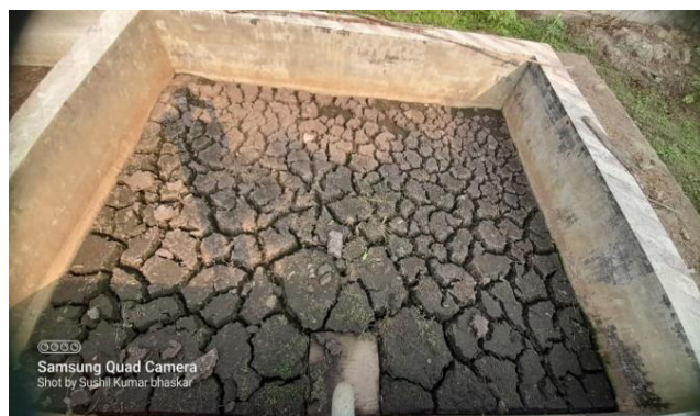
Fig. 14. Sludge Drying Bed Source-Northern Eastern Railway Gorakhpur)
