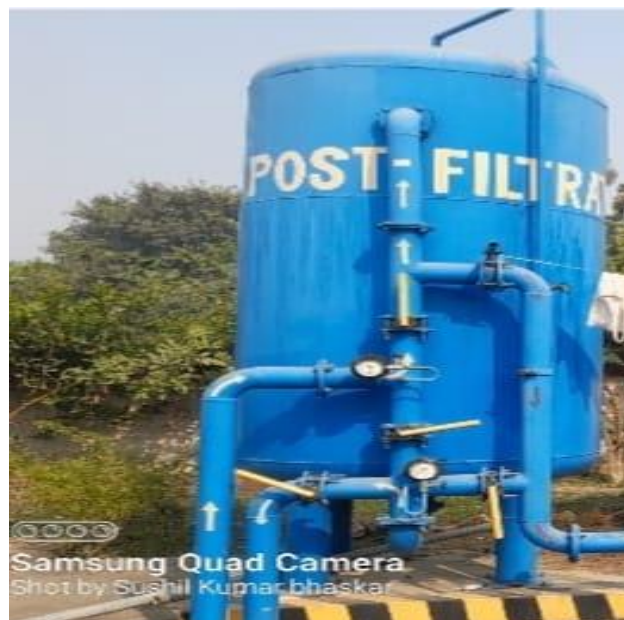
Fig. 9 Secondary Filtration Process (Source-Northern Eastern Railway Gorakhpur)
