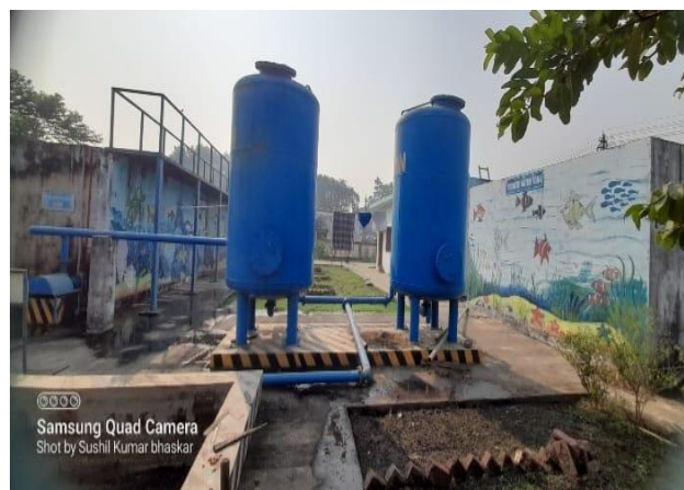
Fig. 10. Secondary Filtration Process (Source-Northern Eastern Railway Gorakhpur)
